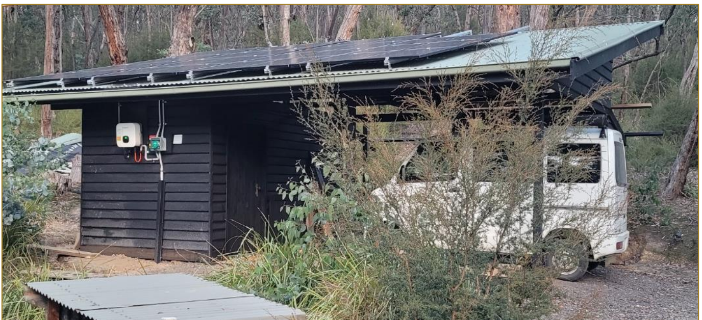
Sean's solar set-up on the roof and his EV mini van in the garage.
